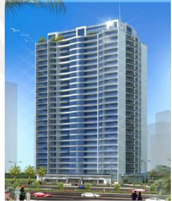
GLOBAL GOLF RESIDENCE - 2 Dubai Sports City, Dubai (05 Elevators)
