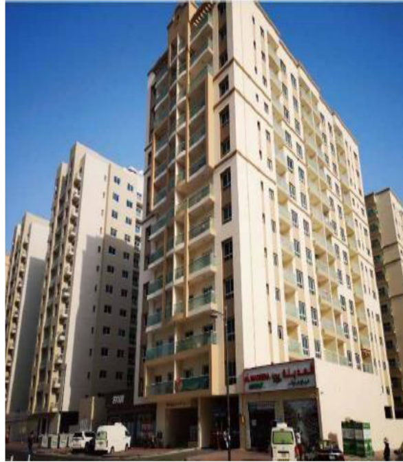
BIN JUMA RESIDENCE Al Nadha – 1, Dubai (06 Elevators)
