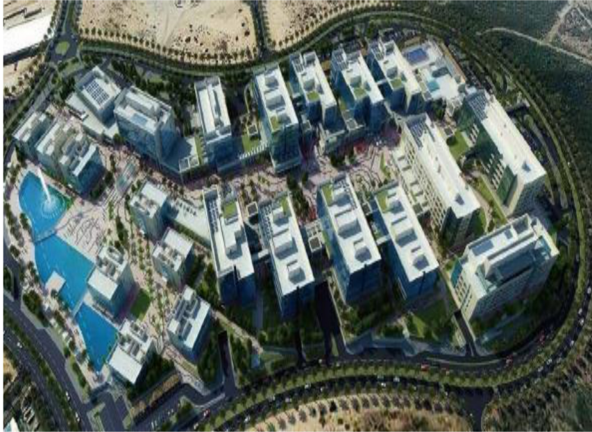
DUBAI DIGITAL PARK Dubai Silicon Oasis, Dubai (72 Elevators and 10 Escalators)
